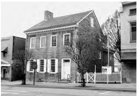
143 South Main Street in Washington, Pa. (right) anchors the block with the historic Bradford House (below). In 2011–12, The Landmarks Development Corporation was hired to manage the repointing of the stone work, replacement of the wooden shake roof, and painting of the trim.
