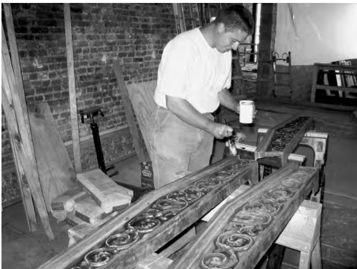
Left: There are 78 windows in the three buildings comprising Market at Fifth. The ceilings in the apartments are about 12 feet high. Right: The cast-iron window hoods were taken down, stripped, repainted, and reinstalled. “When one window hood cracked, we made a new one—and it’s impossible to figure out which is the new one,” said Paul Boggeman.
