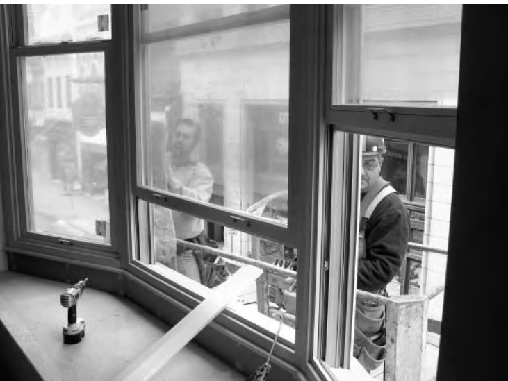
Left: There are 78 windows in the three buildings comprising Market at Fifth. The ceilings in the apartments are about 12 feet high. Right: The cast-iron window hoods were taken down, stripped, repainted, and reinstalled. “When one window hood cracked, we made a new one—and it’s impossible to figure out which is the new one,” said Paul Boggeman.
