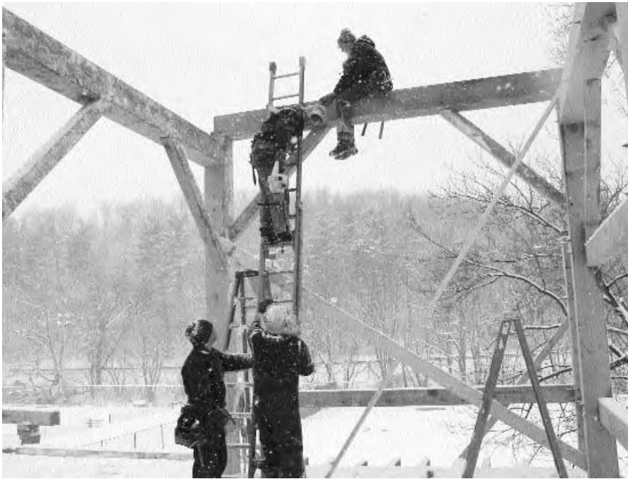
December 14, 2004: Amish Timber Framers of Doylestown, Ohio, at work amidst snow squalls. The timber frame will be covered by boards and battens, and the roof will be covered with recycled material of simulated shakes. The barn will be completed by the summer of 2005.
