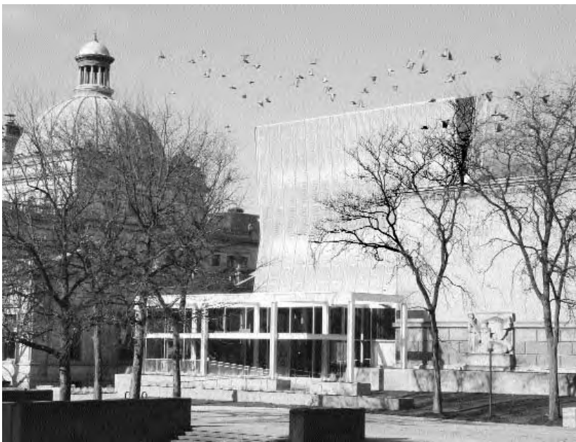
The expanded Children’s Museum of Pittsburgh on the North Side connects 19th and 20th century landmarks with a three-story 21st-century structure whose façade of hinged, polycarbonate squares ripples in patterned waves like water when it’s windy. The rotunda space (right) has been beautifully restored and adapted as an art center and exhibit area.
