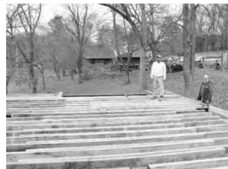
The timber frame was set on a concrete block foundation that will be faced in stone.
