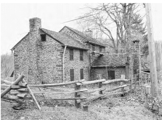
Inappropriate aluminum gutters were removed from the Oliver Miller stone manse, and wooden "V-shaped" gutters were installed as part of the grant project.
