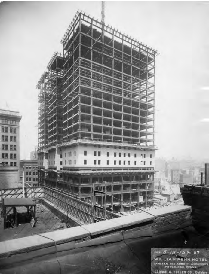
Left: May 15, 1915—The steel frame of the William Penn Hotel with the terra cotta facing being installed. Above: The splendor of the renovated lobby in 2003.
