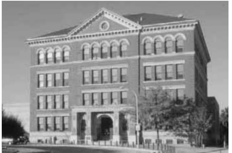
Allegheny, 810 Arch Street, North Side. Frederick J. Osterling, 1904; M. M. Steen, 1936 (Historic Landmark Plaque, 1992)
