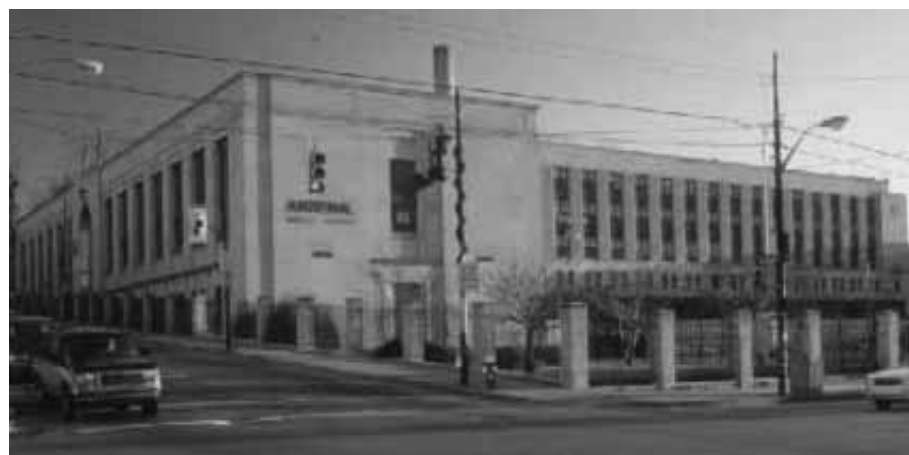
Arsenal, 3900 Butler Avenue, Lawrenceville. Schwab, Palmgreen & Merrick, 1932; M. M. Steen, 1939
