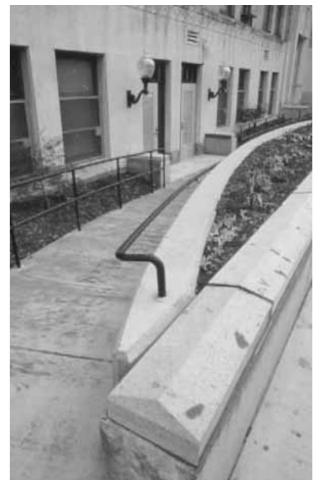
In 2000, Landmarks presented an Award of Merit to the Board of Public Education for the sensitive design and installation of a handicapped-accessible entrance to the 1936 Allegheny school building.
