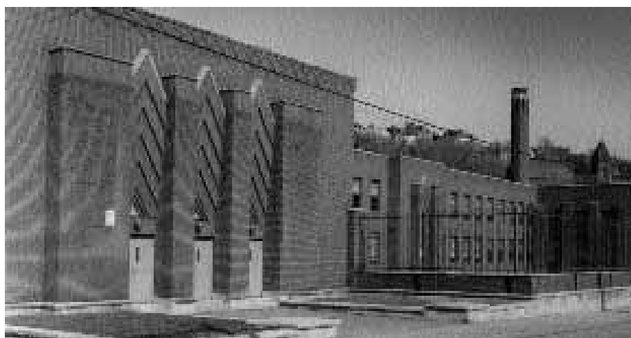
Schiller, 1018 Peralta Street, East Deutschtown. Edward J. Weber (M. M. Steen, Supervising Architect), 1939
