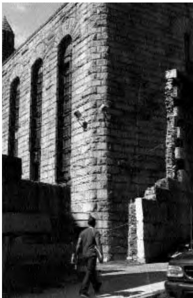
The gap in the Fifth Avenue jail-yard wall, to become an archway. Trucks and the public will both pass through, the latter to a park area. Note the thinness of the stone facing—about eight inches at the top—and the brown backup brickwork. The bulging "basket" bars of an Osterling addition are still in place.
