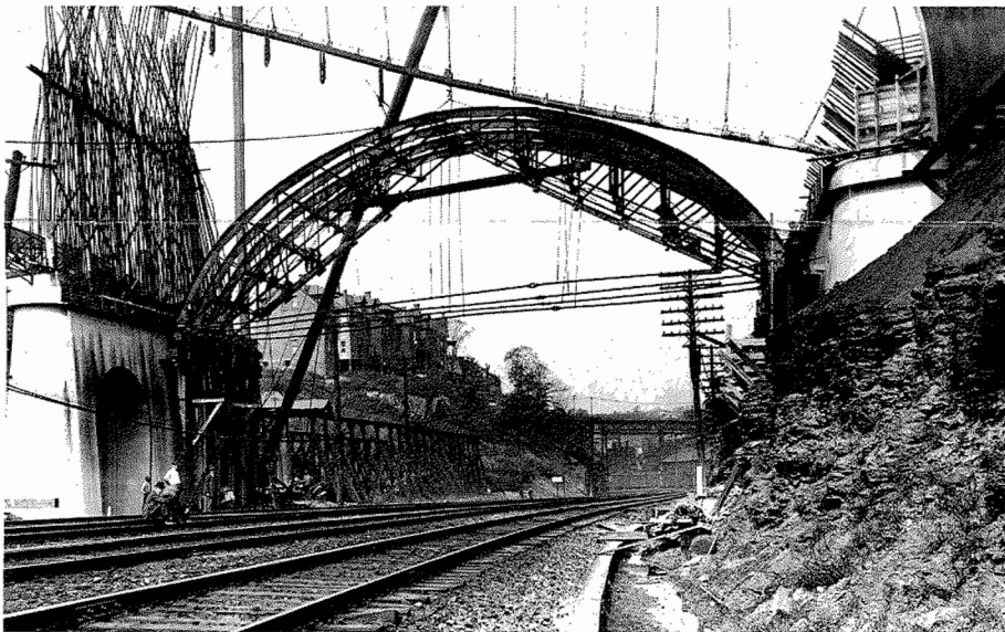
In September 1912, the project to carry Atherton Avenue over the Pennsylvania main line had gone this far: arch falsework that looks very light, sprays of reinforcing rods.
