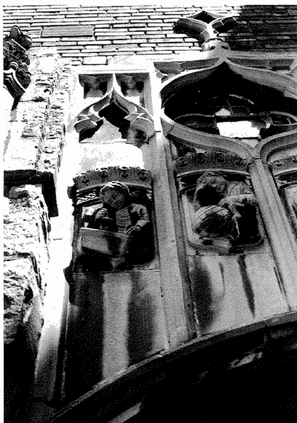
The greater part of St. Philip's School in Crafton also was built in 1927, with warm-toned rock-faced sandstone below and rich red brick above. The masonry is unusual in that, not only is the sandstone random ashlar—squared in various dimensions and jigsaw-puzzled together—but so is the brickwork. You think of brick as a modular material, easily assembled, but Bertram Goodhue, for instance, at St. Bartholomew's Church in New York, used labor-intensive fitting-together of differently dimensioned bricks in order to get a varied, random pattern; and so it is here. Another Weber design, most likely.
