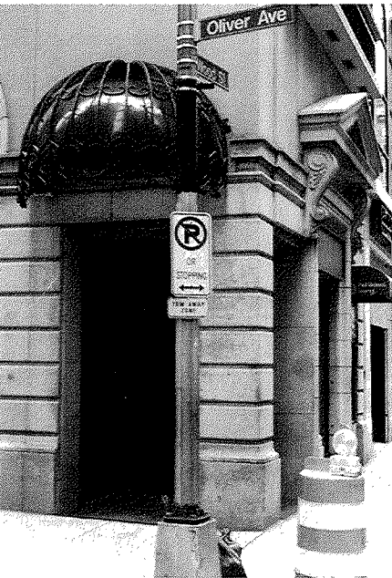
The granite lower story of the Third National Bank. The original upper wall surface was pale warm-gray Roman brick. The canopy and the sign over the pediment are additions.
