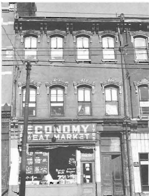
1705 East Carson Street as it used to be ...
