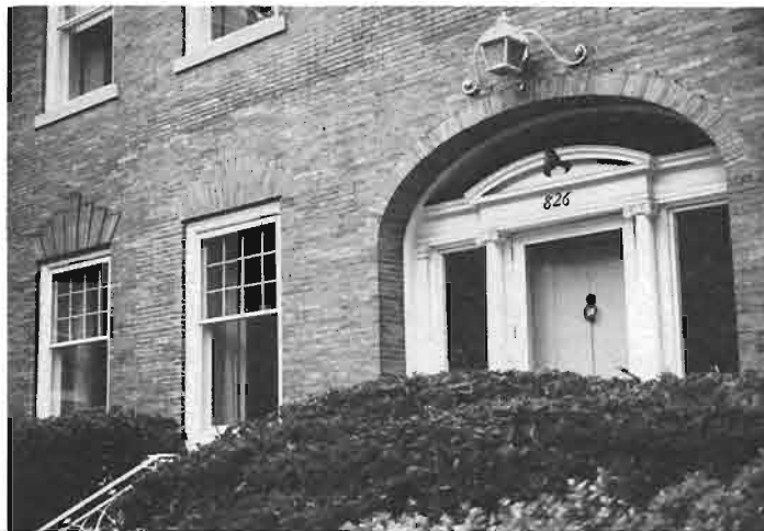
Above: When it was removed, the gap in the face brick where the porch roof met the wall was carefully filled. Only the fact that the outer arches are rusticated and the others are not leads one to suspect the previous existence of a porch.
