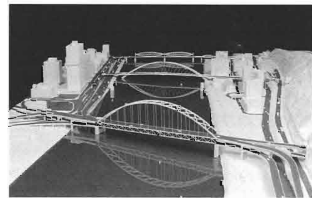
How the basket-handle arch would look. In town the bridge "touches down" near the end of Market Street.
