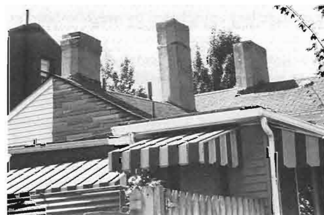
A South Side roofscape.
