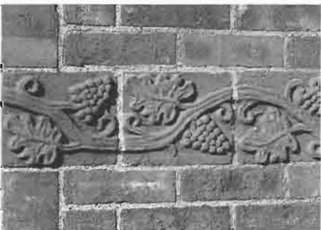
The reveals of the new transept doorways have molded terra cotta.
