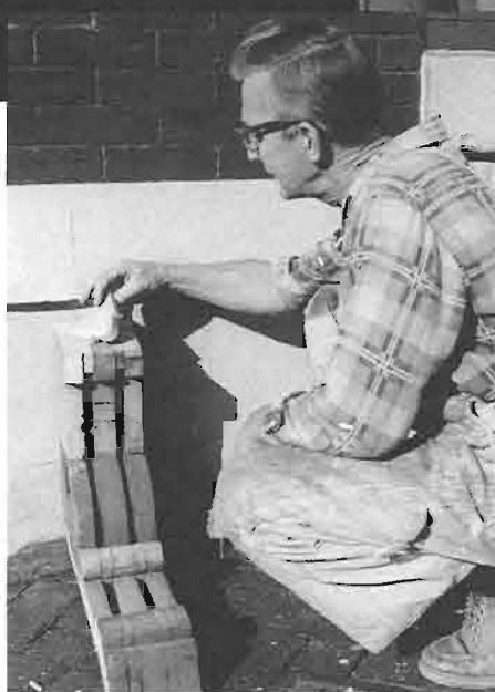
Inset, top left: 1219 Buena Vista Street being cleaned. A Resaca Place doorhead; Warren Schweitzer restores a cornice bracket.
