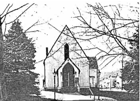
P St. Paul's Baptist Church (1874) in Oakmont is a rare Gothic Revival design of the simplest variety, designed by William Kerr.
