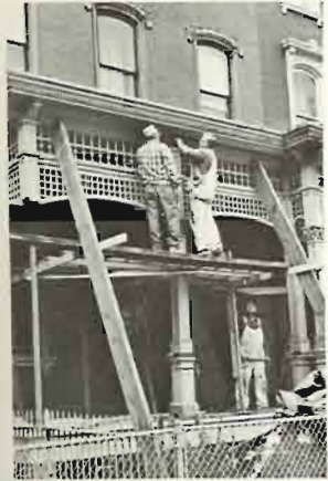
The PHLF work crew under the direction of Warren Schweitzer (upper right) restores the wooden front porch of 404 W. North Avenue in the Mexican War Streets. The porch floor had pulled away from the building and had to be pushed back and anchored into place.
