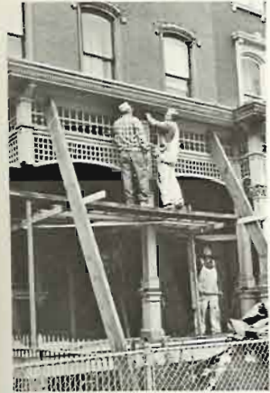
The PHLF work crew under the direction of Warren Schweitzer (upper right) restores the wooden front porch of 404 W. North Avenue in the Mexican War Streets. The porch floor had pulled away from the building and had to be pushed back and anchored into place.
