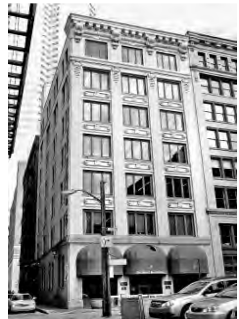
Hartley-Rose Building (Hartley-Rose Belting Company Building) 425–427 First Avenue, Downtown Edward Stotz; 1907 Donor: First Avenue Partners; 1983 National Register of Historic Places; Historic Landmark Plaque
