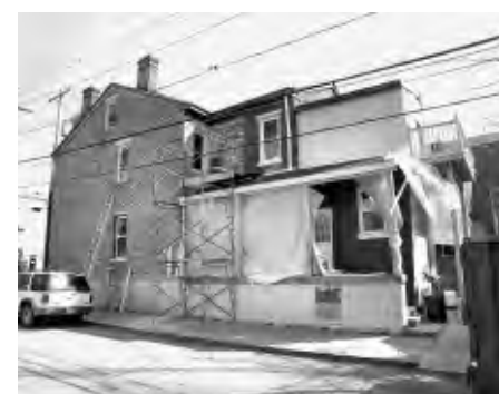
Progress at 182 36th Street, Lawrenceville, as of March 2012
