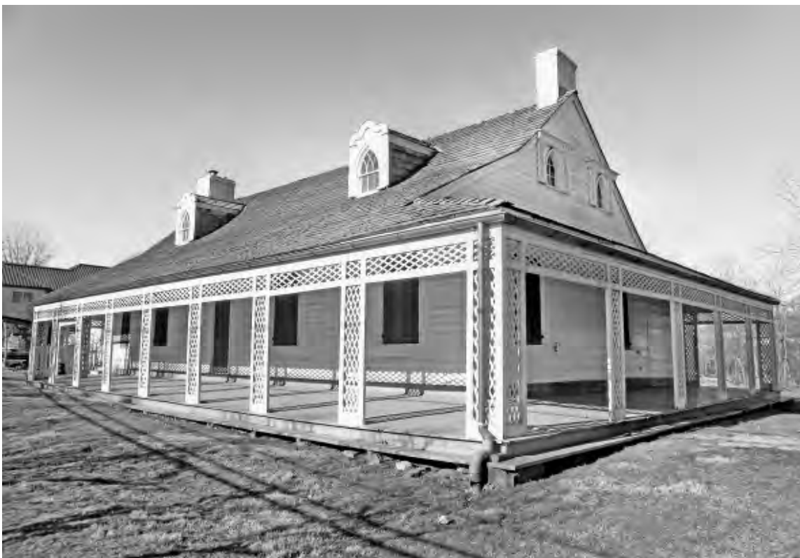
Neville House (Woodville Plantation) 1375 Washington Pike, Bridgeville C. 1785; additions and alterations Neville House Associates, Inc.; 2007 National Historic Landmark; Historic Landmark Plaque
