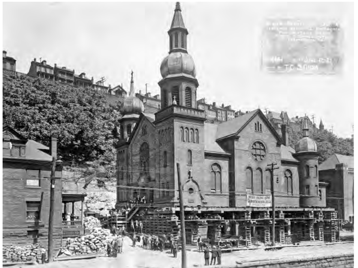
In 1921, the John Eichleay Jr. Company moved St. Nicholas Church, designed in 1901 by Frederick Sauer, to a new foundation further away from the Allegheny River to allow for road expansion. The church rectory, on the left side of the photo, was also moved back to a new foundation in the shelf excavated from Troy Hill. The Catholic Diocese closed the church in 2004 and the building is now vacant (see Advocacy , page 8).
