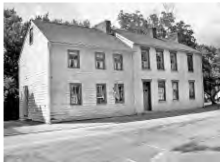
John C. Plumer House 131 Water Street, West Newton Borough 1814, addition c. 1846 Donor: Mon Valley Initiative; 2011 National Register of Historic Places
