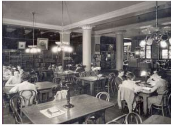
First floor view, c. 1900
