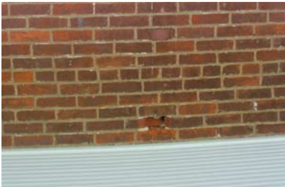
Repair broken brick in rear porch area.
