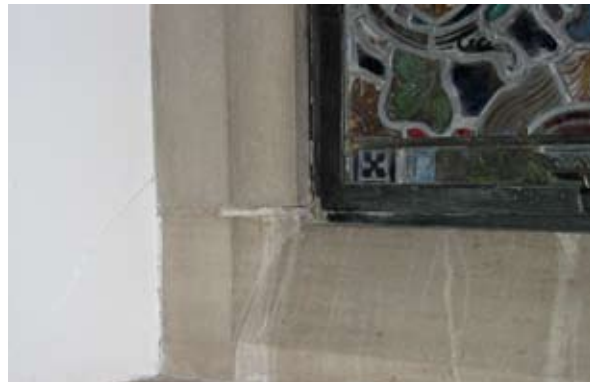
Check stained glass for possible water infiltration around fenestrations.
