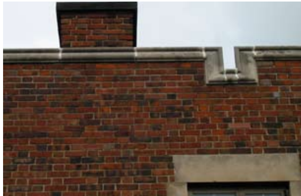
Seal joints in capstones and mortar with materials of original colors and size.
