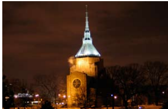
The upper spire has been lighted in a cool metal halide lamp while the lower building is lighted in a warm high pressure sodium vapor light
