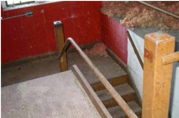
Reattach the top section of railing to stairs.
