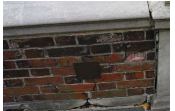
Repair spalling brick at terrace wall.
