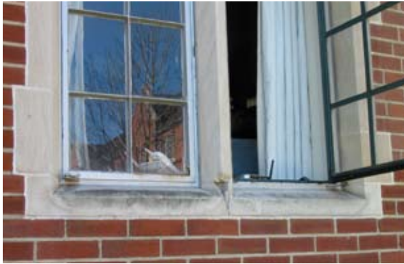
Repair stone at windows as needed.
