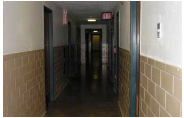
Check the luminance using a light meter to determine safe lighting needs.
