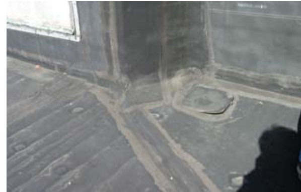
Repair rubber roof patches
