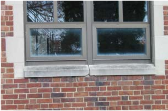
Repair sills and joints as needed.
