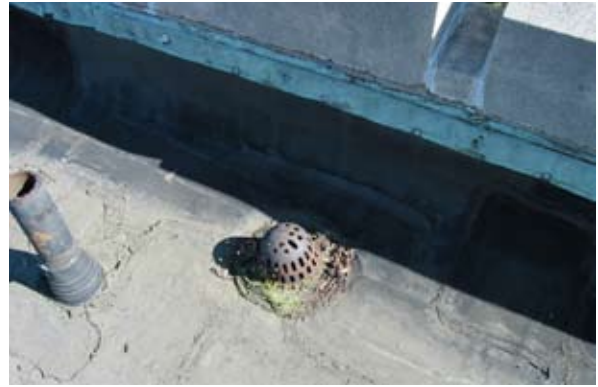
Caulking of the capstones along the parapet walls as needed.
