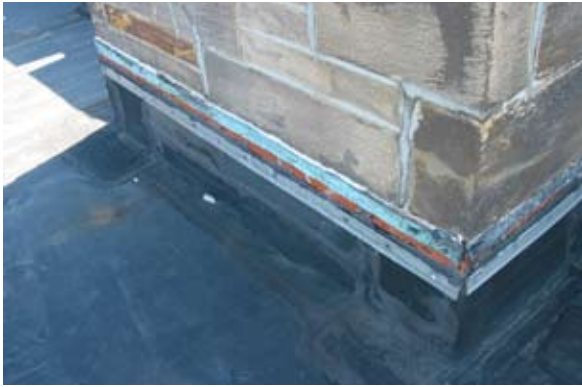
Check termination bars along parapet wall for watertight seal.
