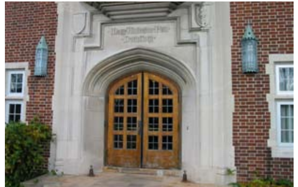
Repair and refinish wooden doors and trims.
