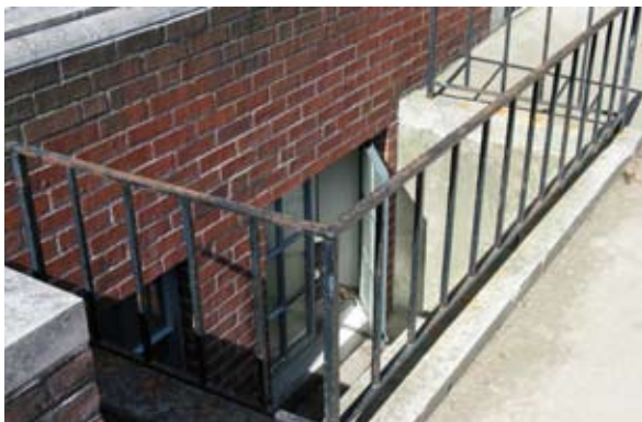
Paint iron railings as needed.
