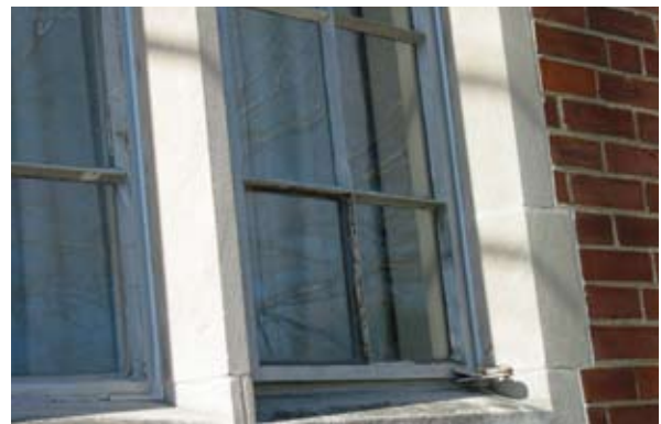
Glaze windows and paint as needed.
