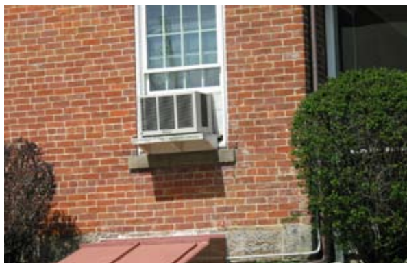
Repoint masonry as needed to match existing.
