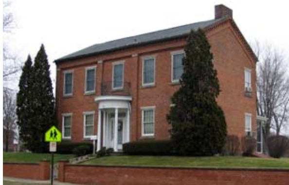
When replacing the existing roofing, consider returning to slate, or slate reproduction in lieu of asphalt shingles.
