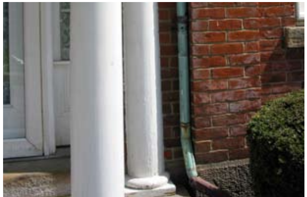
Scrape, prime, and repaint exterior wood columns and trim.
