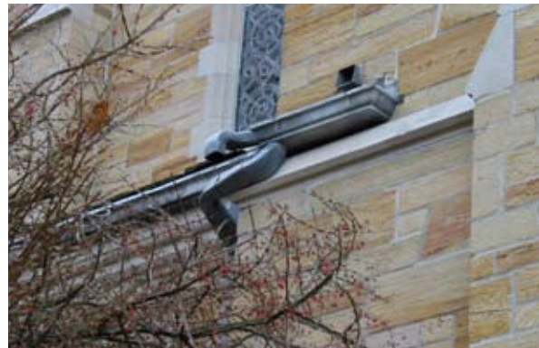
Reattach downspout and elbows.
