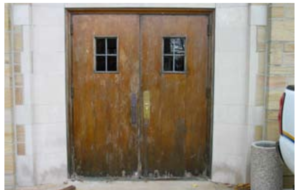
Repair and refinishing of the exterior wooden doors. Install original door hardware where missing.
