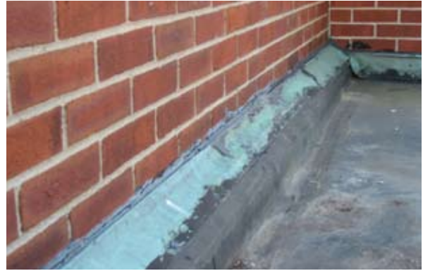
Seal flashing at mortar joint.
