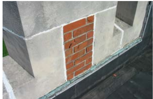
Repair spalling red brick at parapet wall.
