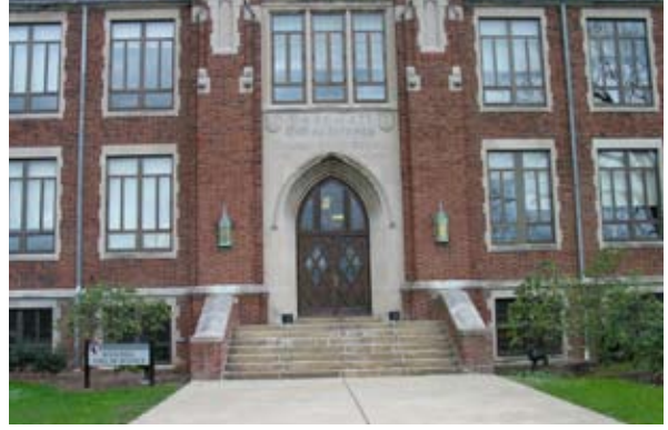
Add iron handrail at entry stairs to match existing ironwork on campus.
