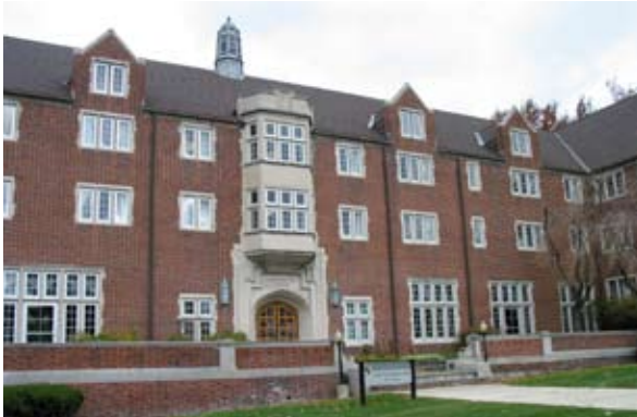
Clean and point masonry as needed.
