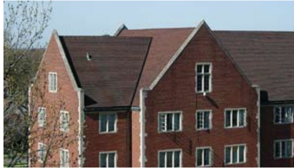
Roof covering example
