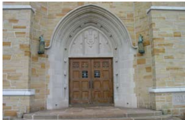
Refinish all wooden doors. Consider handrails at entry stairs matching existing ironwork around campus.
