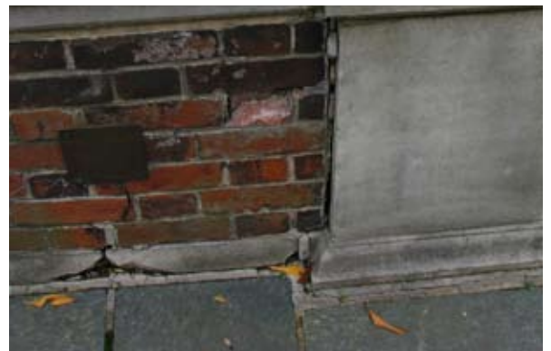
Repair patio stone.
