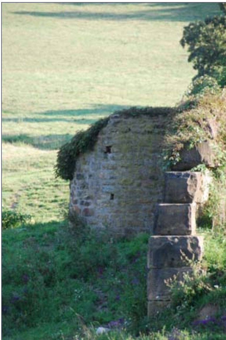
#802068—100 Covered Bridge Rd., Burgettstown, Smith Township Washington County
