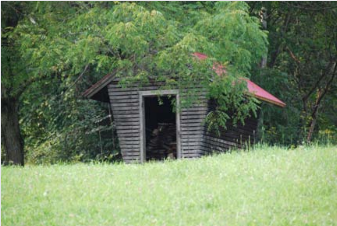
#802093—2194 Reisling Rd., McDonald, Cecil Township, Washington County
