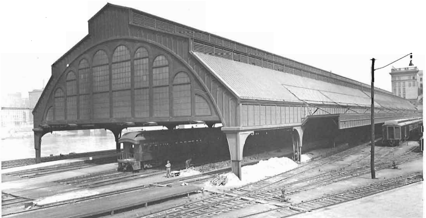
BELOW—The train shed with the addition of 1911. Photo 1916. OPPOSITE ABOVE—The Edwardian Elegance of the Grand Concourse in 1901. OPPOSITE BELOW—The P&LE freight yards with the Central Warehouse (Shovel Building) and the Freight House c. 1916. Photos courtesy P&LE.
