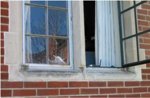
Repair stone at windows as needed.
