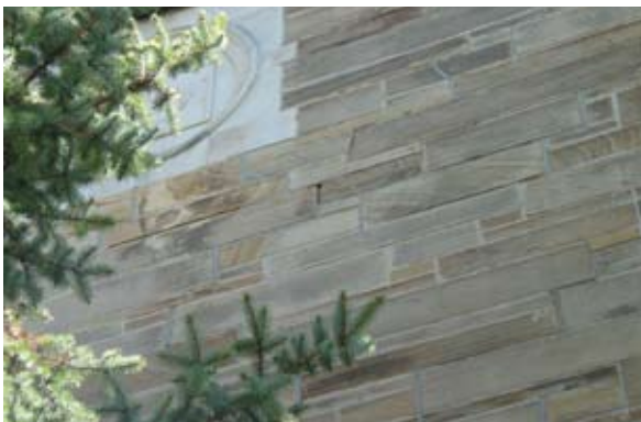
Repair stone and mortar joints as needed. Match color and texture.
