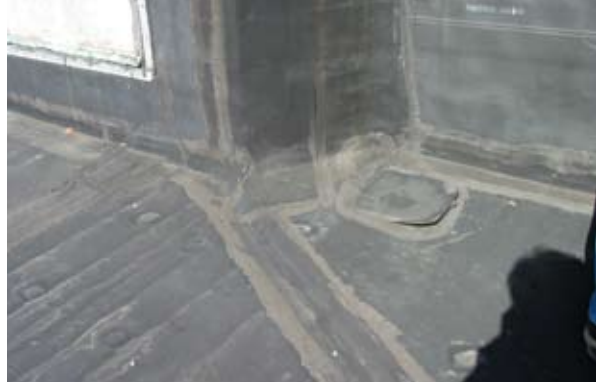
Repair rubber roof patches
