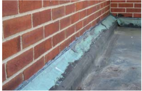
Seal flashing at mortar joint.
