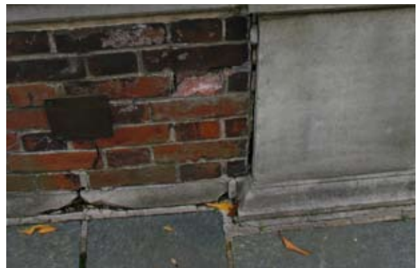
Repair patio stone.
