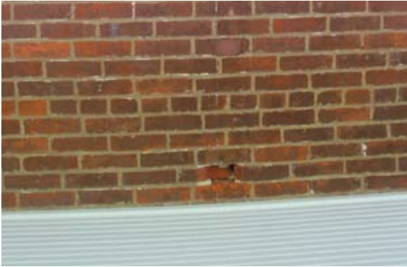
Repair broken brick in rear porch area.
