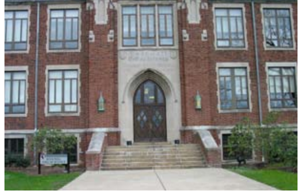
Add iron handrail at entry stairs to match existing ironwork on campus.
