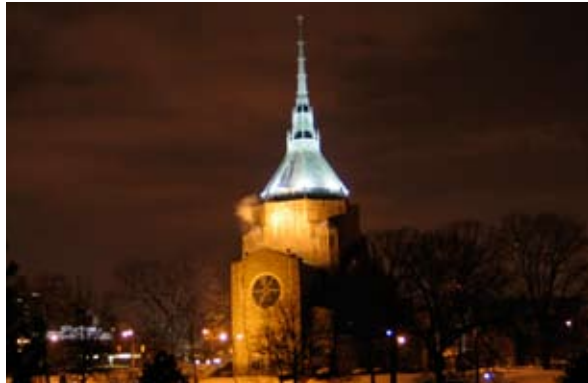
The upper spire has been lighted in a cool metal halide lamp while the lower building is lighted in a warm high pressure sodium vapor light
