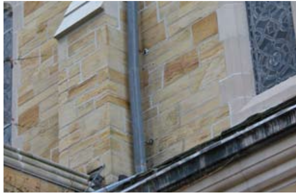
Reattach downspout and elbows.
