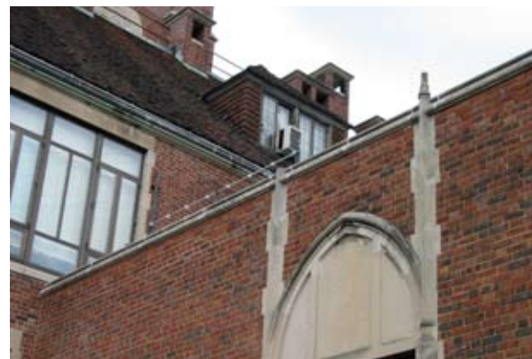
Test clean masonry in inconspicuous spot before doing entire structure.
