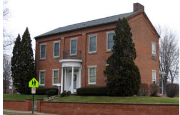
When replacing the existing roofing, consider returning to slate, or slate reproduction in lieu of asphalt shingles.
