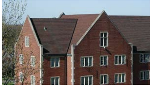
Roof covering example
