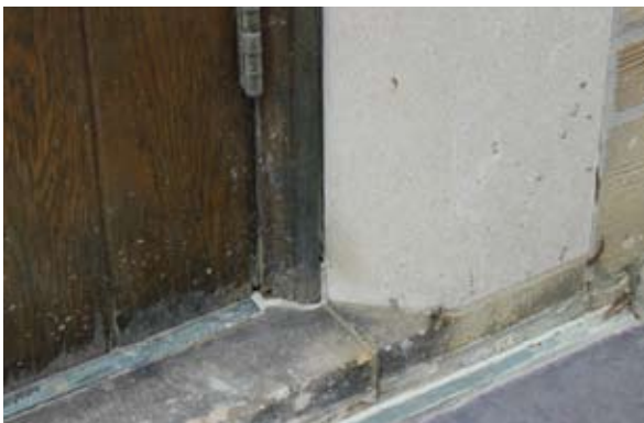
Repair and refinishing of the exterior wooden doors. Install original door hardware where missing.
