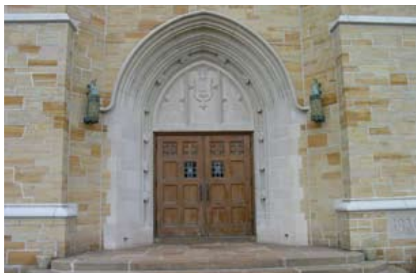
Refinish all wooden doors. Consider handrails at entry stairs matching existing ironwork around campus.
