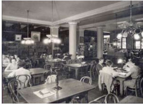
First floor view, c. 1900
