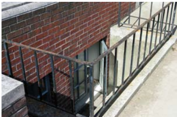
Paint iron railings as needed.
