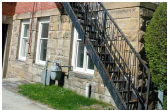
Painting of the fire escape on the east side.
