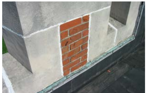
Repair spalling red brick at parapet wall.
