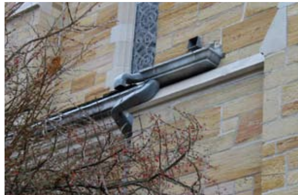
Reattach downspout and elbows.
