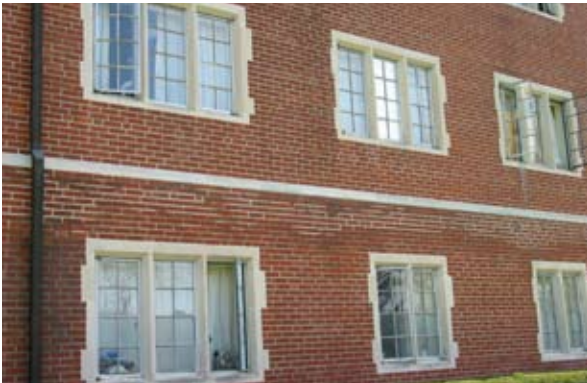
Maintain consistency of size and color of mortar joints.
