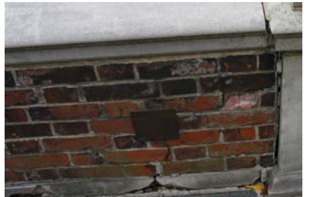
Repair spalling brick at terrace wall.
