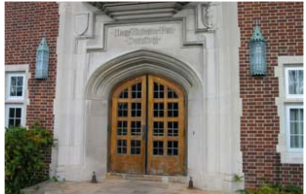
Repair and refinish wooden doors and trims.
