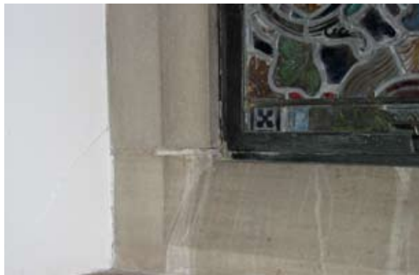
Check stained glass for possible water infiltration around fenestrations.
