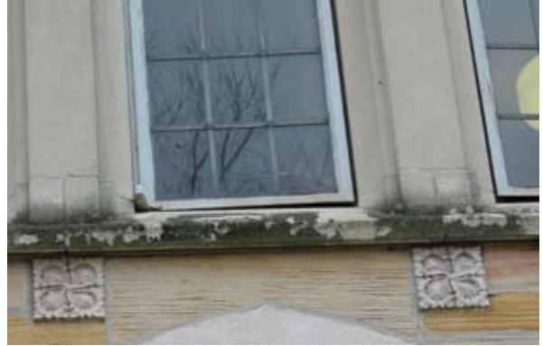
When cleaning masonry, it is suggested to perform a test cleaning prior to the start of work for review and approval to proceed. It is further suggested not to apply waterproof sealants to the exterior of masonry.
