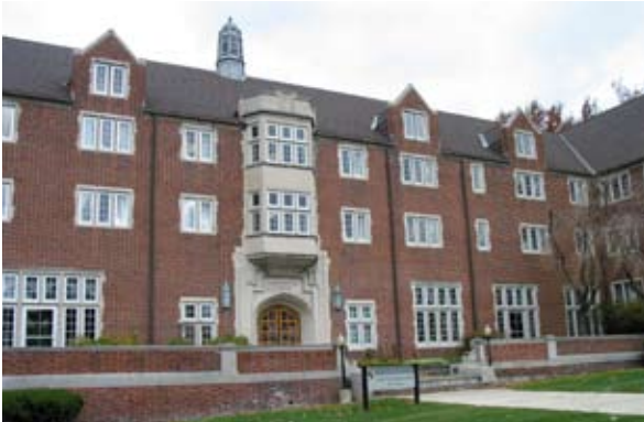
Clean and point masonry as needed.
