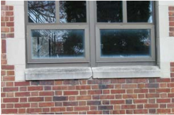
Repair sills and joints as needed.
