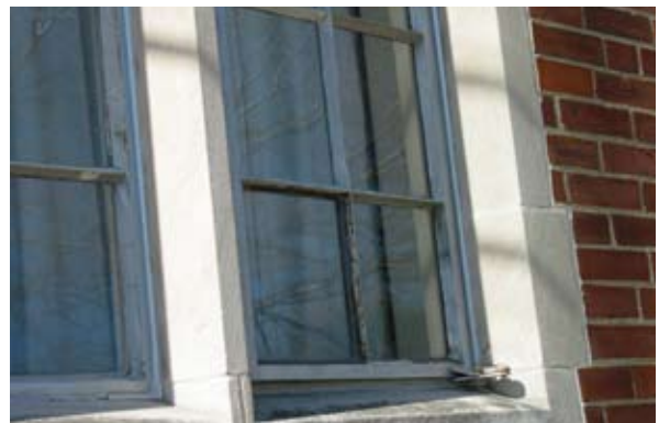
Glaze windows and paint as needed.
