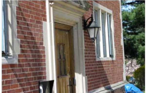
Varnish exterior doors as needed.
